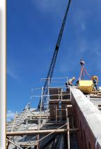
rotted rafters on the nave roof and steeple. The entire church roof was re-decked with 1x4's in order to provide a level, consistent place where upon Vermont slate was hung. The entire steeple structure was rebuilt and reinforced with new lumber. The slate design restored the cross motif on the north and south sides of the nave roof, per the original design when our church was first constructed.
