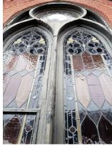
wood frames will be scraped and repaired as needed, before being painted. New ventilated frames and protective glass will be added to those seven windows.
