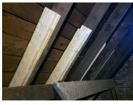
supports, some of which had begun to separate or turn. In other places, extra support was provided to cracked or compromised components by "sistering" new 2 x 8's and micro-laminate beams.
