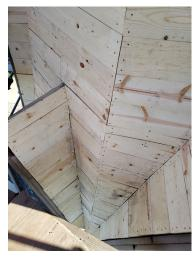
new slate can be attached, new 1x8" lumber is being installed. As of the end of last week, over 350' linear feet of decking was replaced on the steeple gables and hips (right above the
