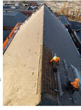
the roof, adding in the longevity of the underlayment and wood decking. Because the slate will be nailed to the battens - at the average of 34 nails per square vs. 390 directly nailed per square through the 40# felt / ice & water guard, there would be many fewer penetrations.
