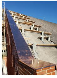
On the nave roof of church, the removal of the clay tile continues. Having removed the numerous layers of tar paper, some rotted  $1 \times 10^{\circ}$  have been replaced on the roof deck. Once
