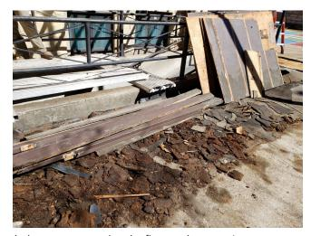
underlayment supporting the five condenser units was disintegrating.
