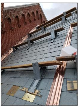
practice of traditional metal and masonry work, copper flashing
