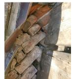
current condition of some of the brickwork behind the roof flashing.
